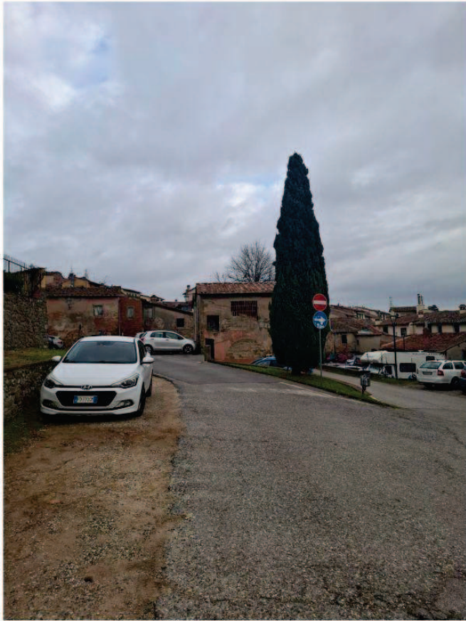
Fig. 8 - lack of accessibility for pedestrian
