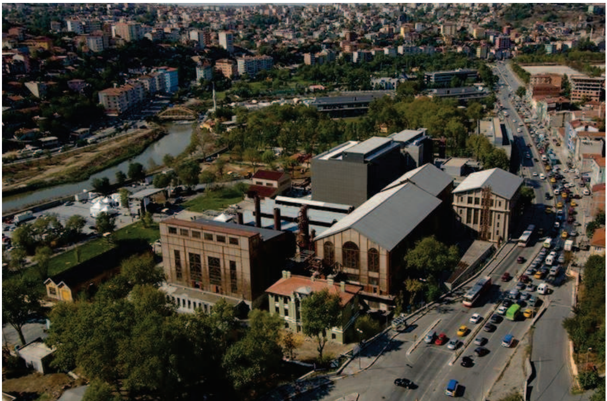
Fig. 24 - The final view of the project
